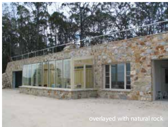
completed structure before render
